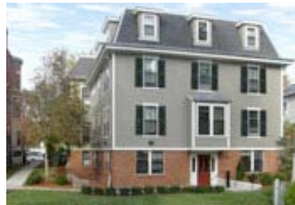
16-18 Wendell Street, Rear View
