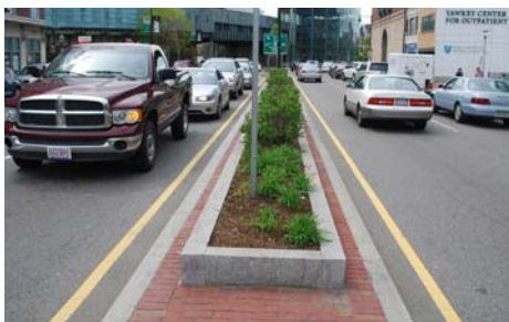
10. Planted Median at High Traffic Street In Boston, Cambridge Street's upgraded medians have reduced jaywalking. The dimensions of this Boston street are similar to the study area stretch of Mass Avenue.
